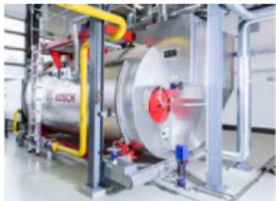
Fig. 61 Condensing heat exchanger
